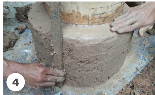
4 Smoothen the walls and measure the right height. There should be a finger sized gap between the wall and the pot.
