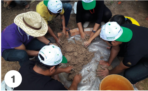
1 Mix clay with some water. Build stove on plastic if you need to move it to another location when ready.
