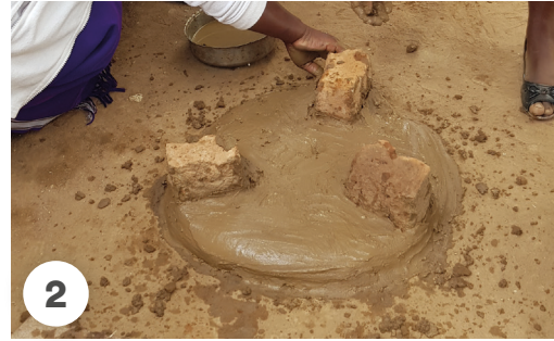
2 Draw a circle the size of your pan on the ground. Lay three bricks equal distance apart on the circle. Start building walls for the stove.
